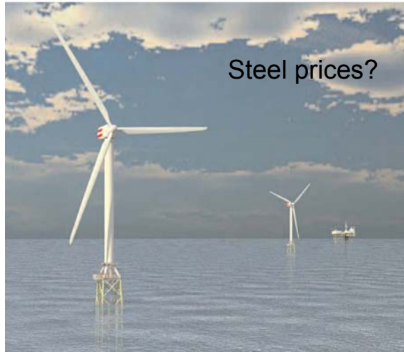
The Beatrice wind farm consisting of two 5 MW wind turbines in 42 m deep water. Source www.beatricewind.co.uk
