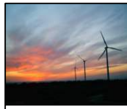
January 2005 Three prototypes installed at Trent Mesa
