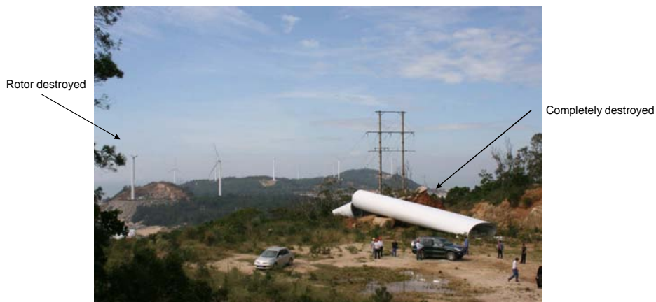
2010, Megi, with 38m/s max 10min wind speed at center when landing, grid on
