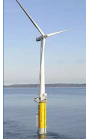
Statoil 2.3 MW Floating Turbine Deployed 2009 - Norway
