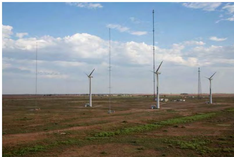
Scaled Wind Farm Technology Facility
