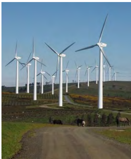
Carballeira Wind Farm - Spain
