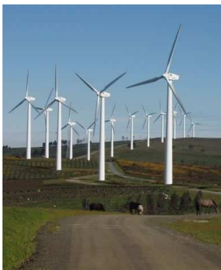
Carballeira Wind Farm - Spain
