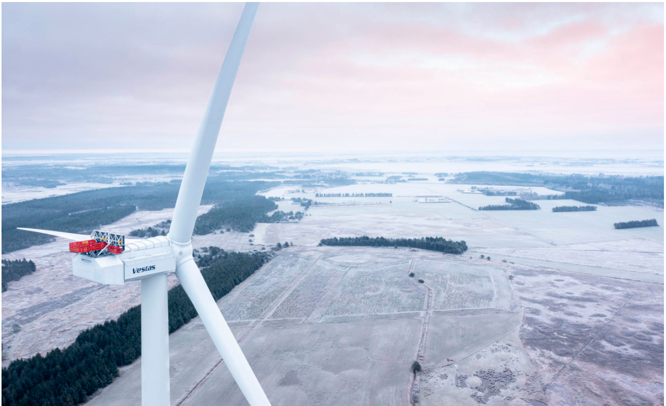
Figure 5. Vestas V236-15 MW wind turbine at Østerild Test Centre
