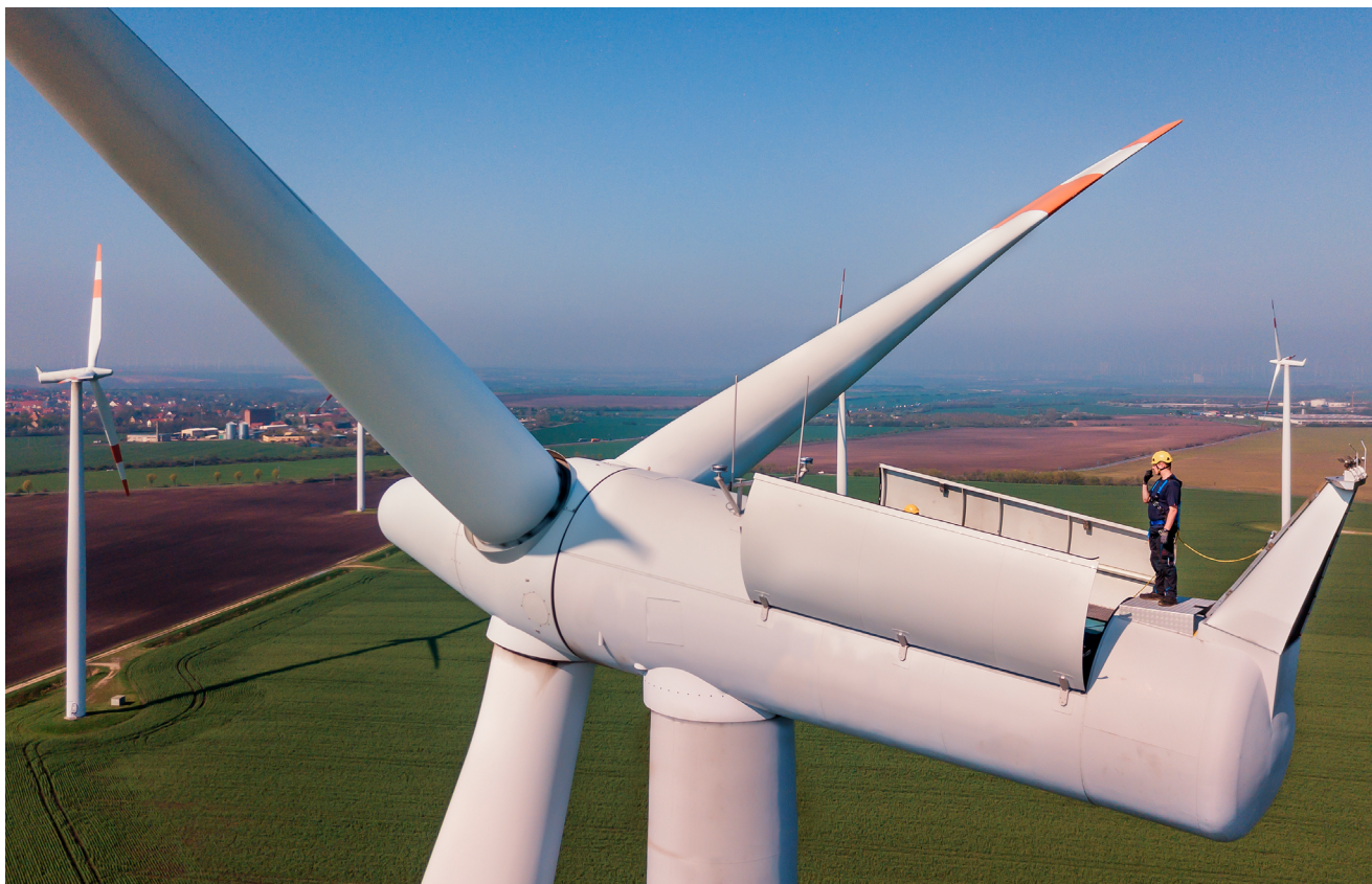
Figure 2. Worker on land-based Wind Turbine. Source: ©Tarnero – stock.adobe.com
