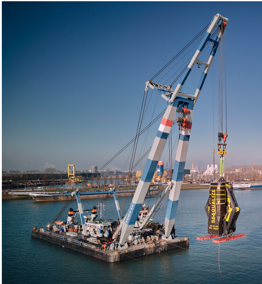
Photo 1: Heave Chief 1100 in the crane of a test vessel in the harbour. (Source: Seaqualize)
