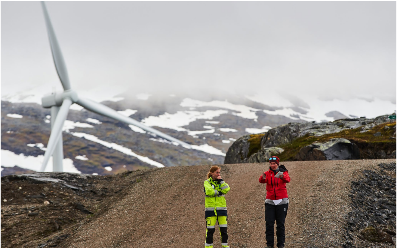
Sørfjord wind power plant #1. Photographer: Catchlight, NVE.
