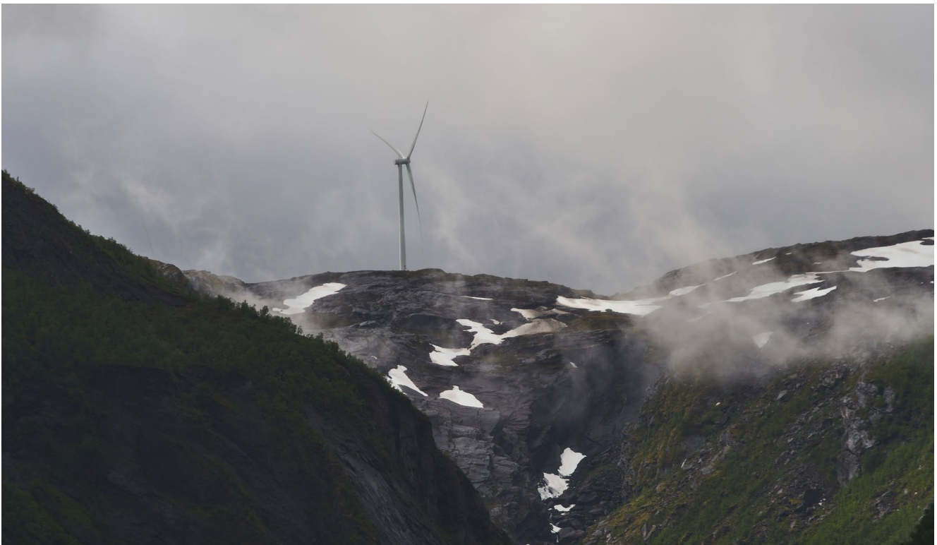
Sørfjord wind power plant #2. Photographer: Catchlight, NVE.
