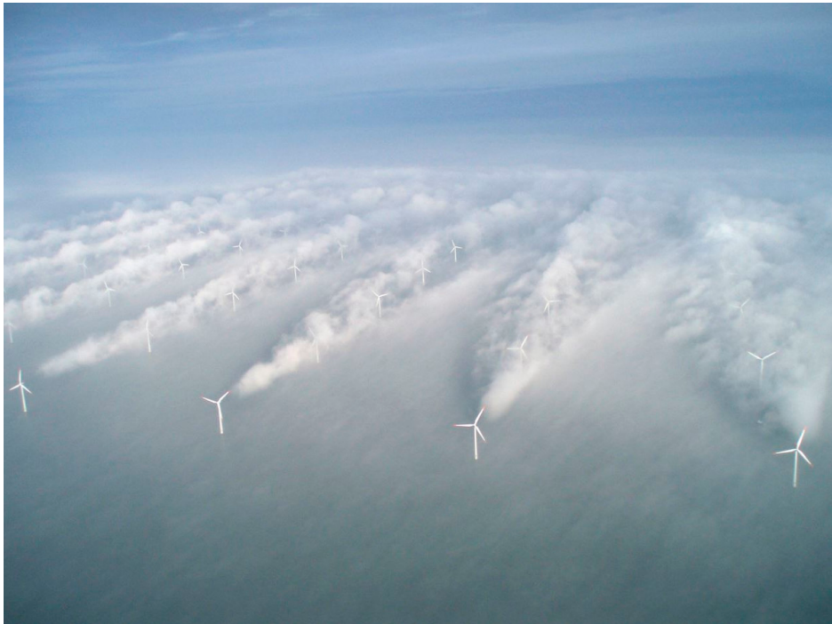
Figure 2. Under dedicated meteorological conditions, the wakes are visible within a wind energy farm. Photo taken on 12 February 2008 at the offshore Horns Rev 1 wind farm, which has a minimum spacing of 7.5 rotor diameters. Graphic courtesy of Vattenfall.
