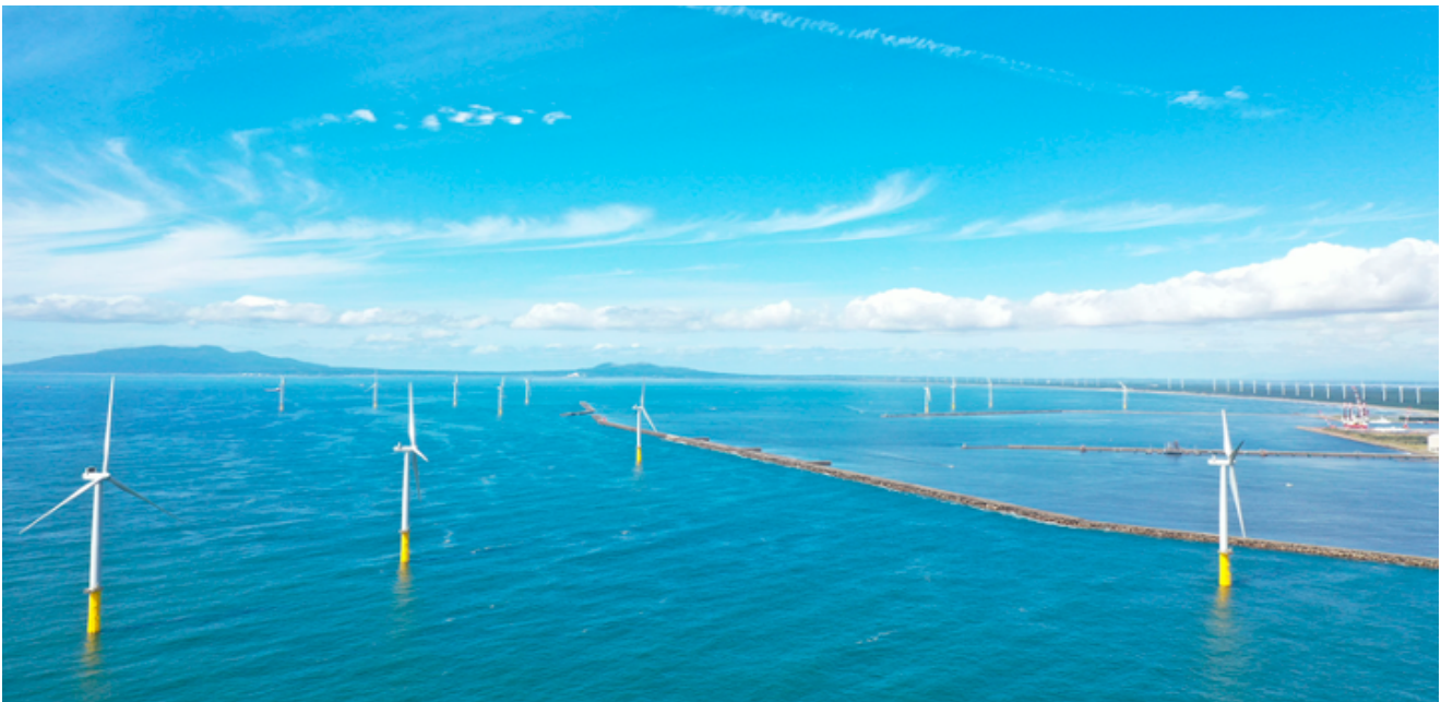
Figure 2: The first large-scale commercial offshore wind farms in Japan. Photo Credit: Akita Port Wind Farm.
