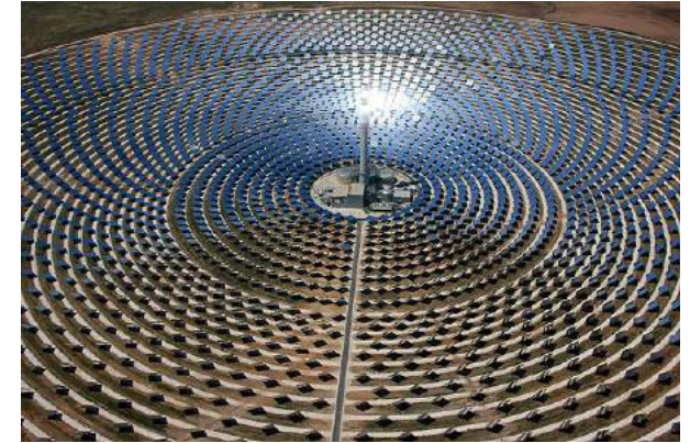
GEMASOLAR power plant, Spain
