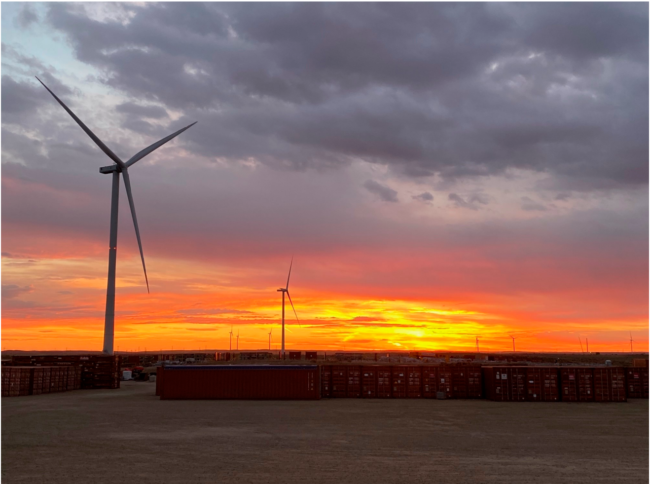
Photo 1: Jenner Wind Projects. Credit: ENERCON Canada Inc.
