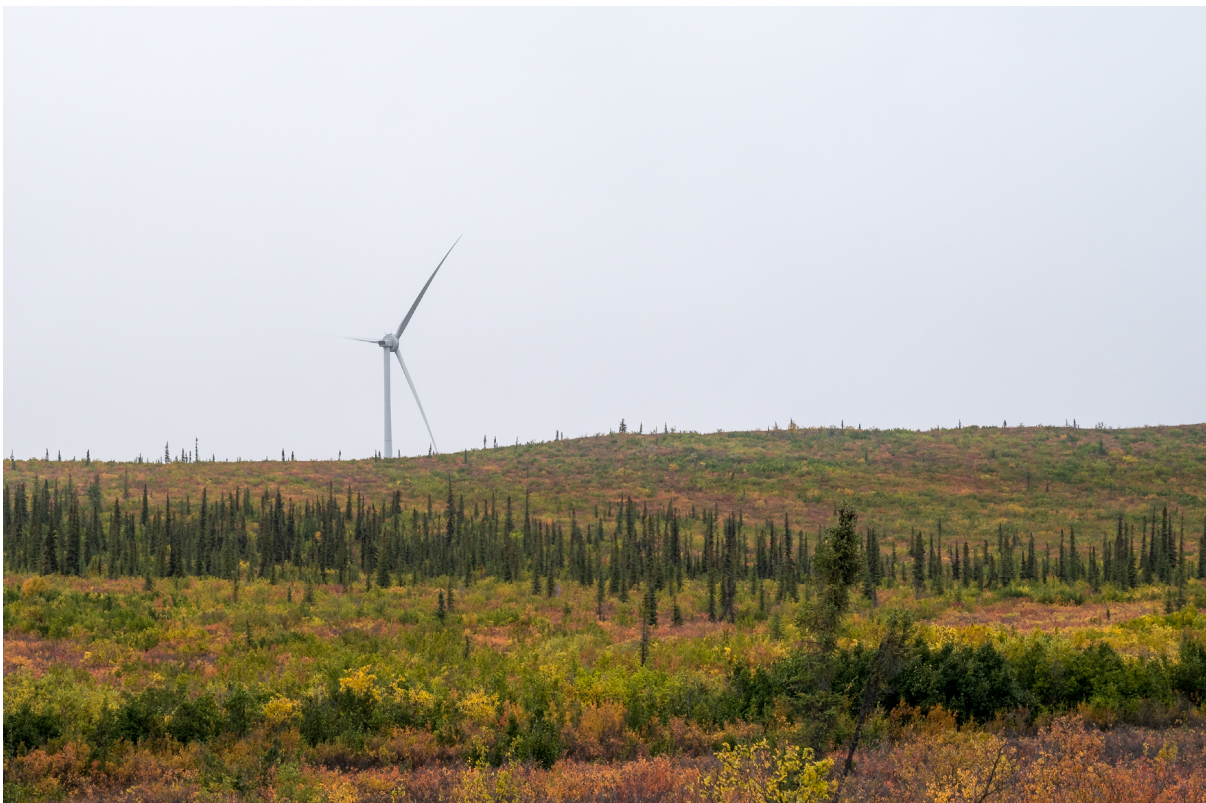
Photo 2: Inuvik Hight Point Wind Project located in Inuvik, Northwest Territories. Credit: ENERCON Canada Inc.
