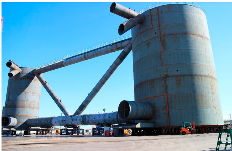
Photo 1: Exterior view of floating foundation mock-up.
