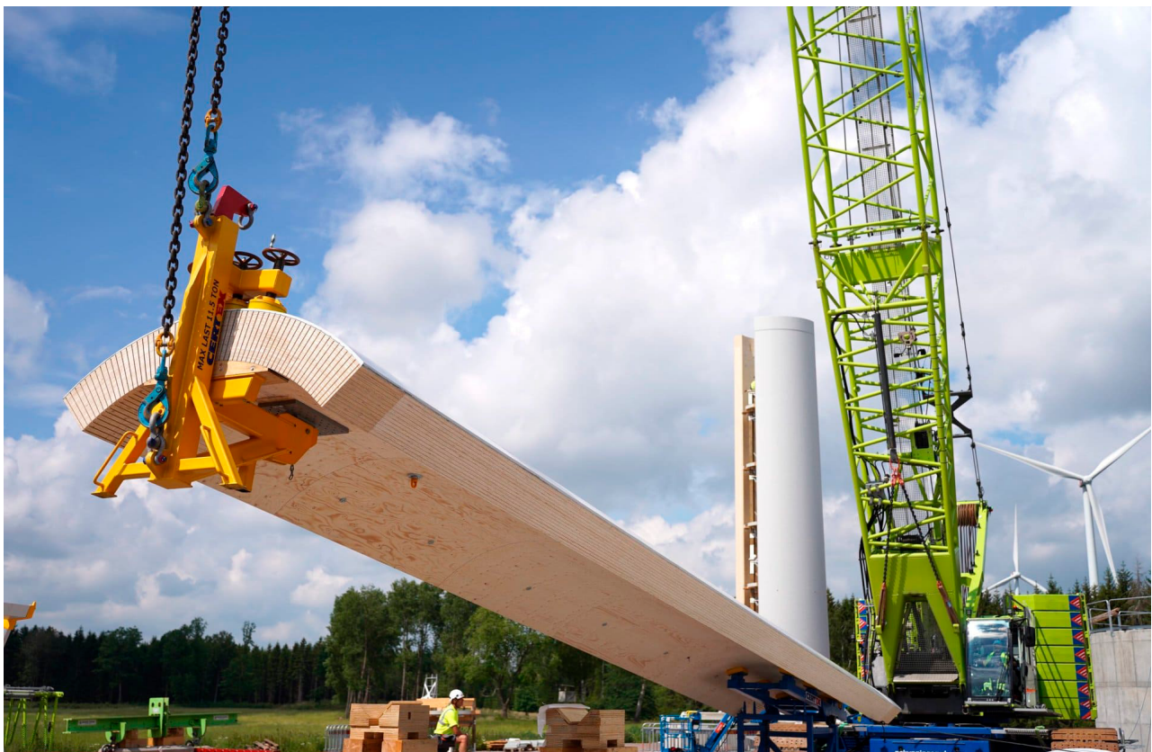
Image 1. Laminated wood tower module. Photo Credit: Modvion.
