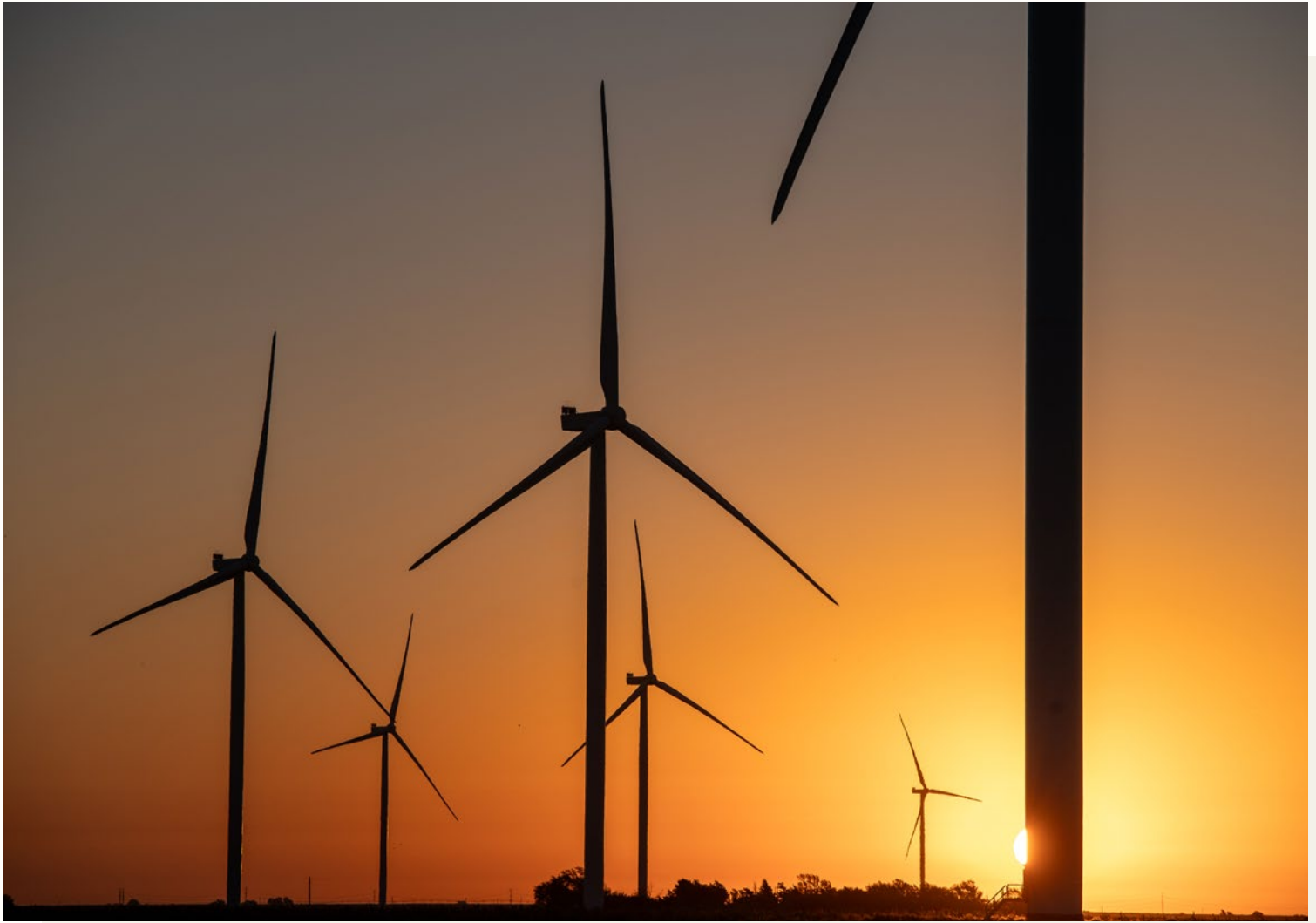
Figure 1: The Iron Star Wind Project, operated by ENGIE North America, is located 5 miles south of Dodge City, Kansas.
